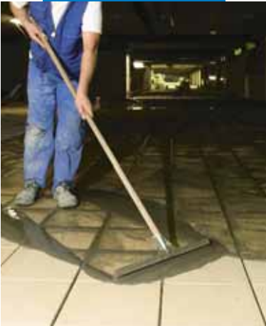
Application of Maxifuga using a rake
