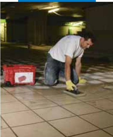
Cleaning surface with Scotch Brite® pad
